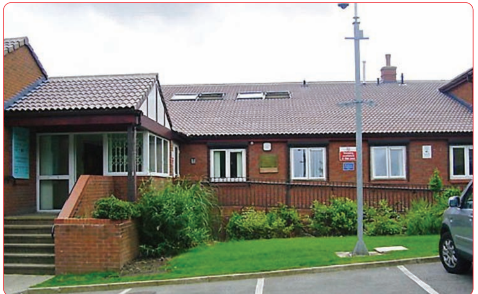
Before and after: Manor Park Surgery has been successfully re-built and re-opened...
